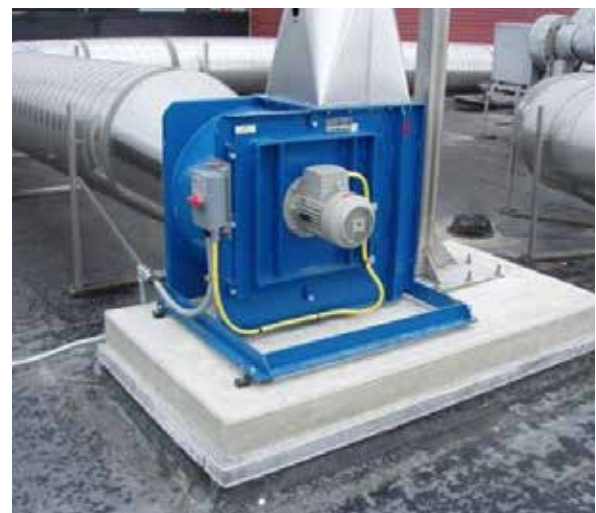
Fan placed on the roof.
